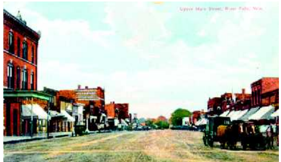
Figure 3. Early Main Street in River Falls.
