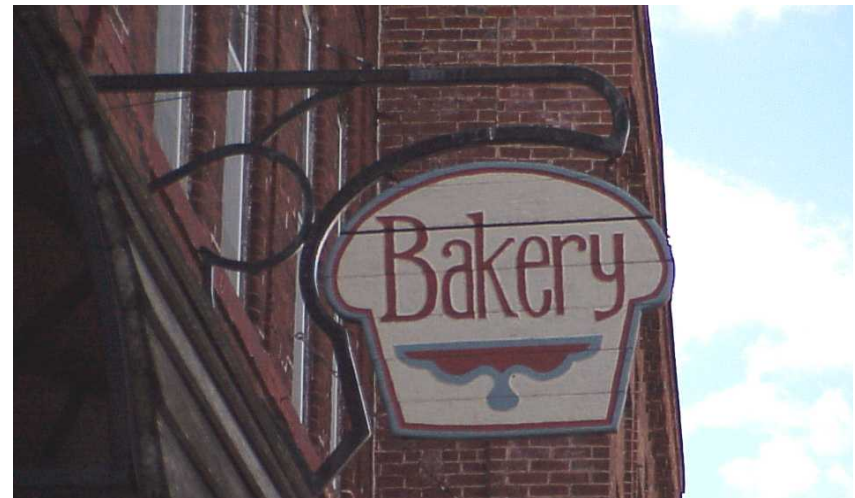
Figure 22. A typical cantilever sign.
